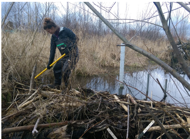
Water levels can be temporarily managed by notching dams. This work requires planning and training to ensure minimal impact to aquatic habitat. MCCA Maintenance Crews are trained to do this work. Call the maintenance office if you think a dam needs attention.
