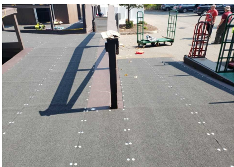
Mill Creek Community Food Bank's rebuilt ramps
