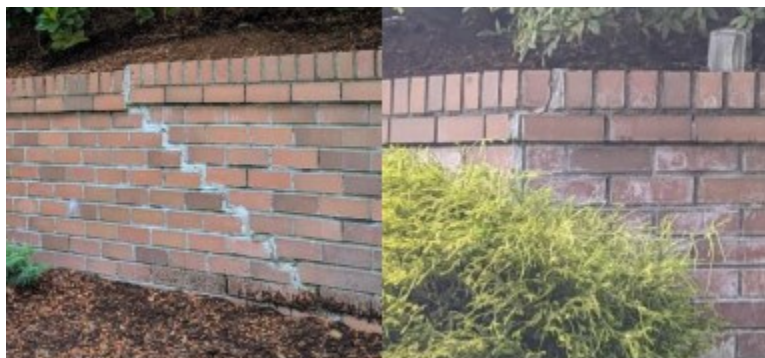
Detail of damage caused by tree
