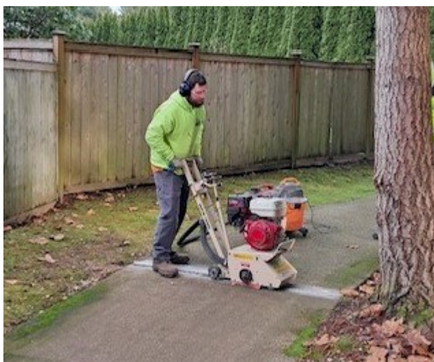
Ryan grinding a potential trip hazard on the trail in Vine Maple
